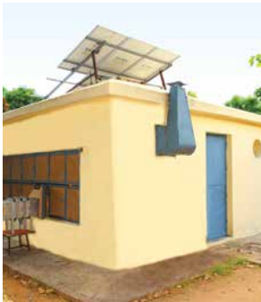
CIPHET evaporative cooled storage
