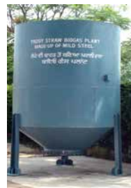
Paddy straw based biogas plant
